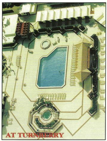
The pool deck and cabanas above were leaking water into the parking garages and apartments located below them. The deck was stripped, and two coats of **R400 RUBBER** embedded in Polyester Reinforcing Fabric were applied to the surface. This system eliminated the leaking problems. The deck was then topped with brick pavers to provide a walking surface.
